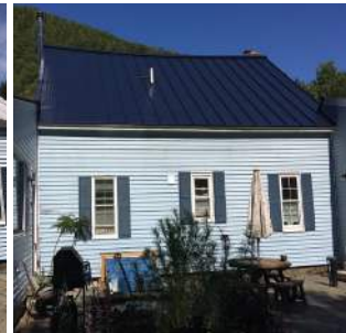
Roof repair, after
